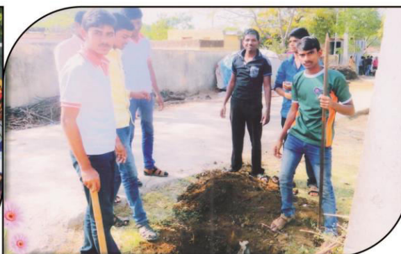
Volunteers digging pits for Tree Plantation in the adopted village.
